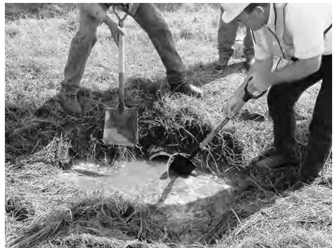
Figure 48. Clearing drainage outlet, Texas SPS-1.
