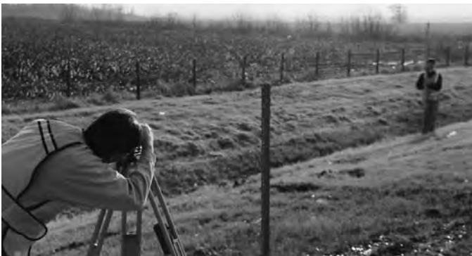
Figure 56. Rod and level measurement of elevation of bottom of drainage outlet pipe at headwall.
