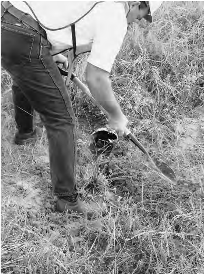
Figure 47. Clearing drainage outlet, Texas SPS-1.
