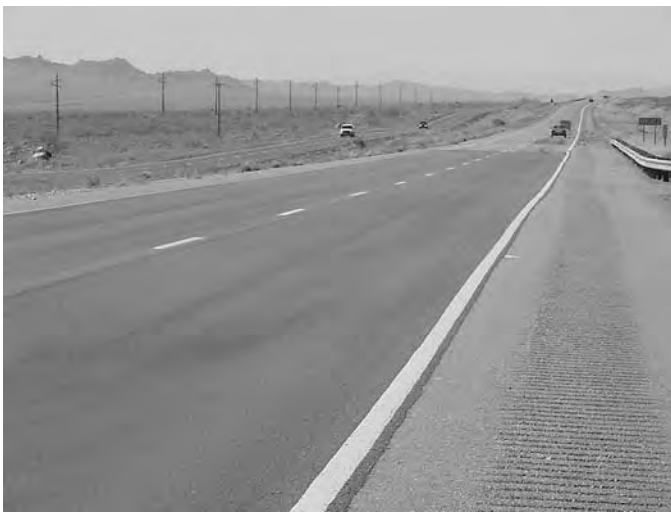
Figure 14. Arizona SPS-1 site.
