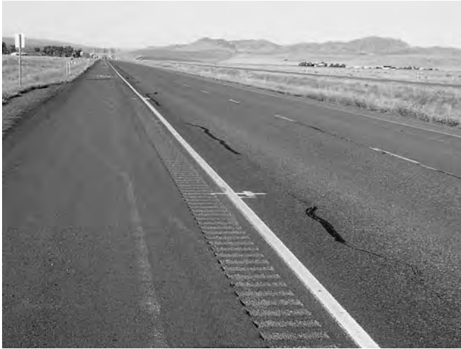
Figure 33. Montana SPS-1 site.
