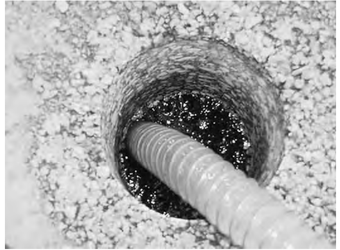
Figure 62. Water inflow from flow meter to PATB.
