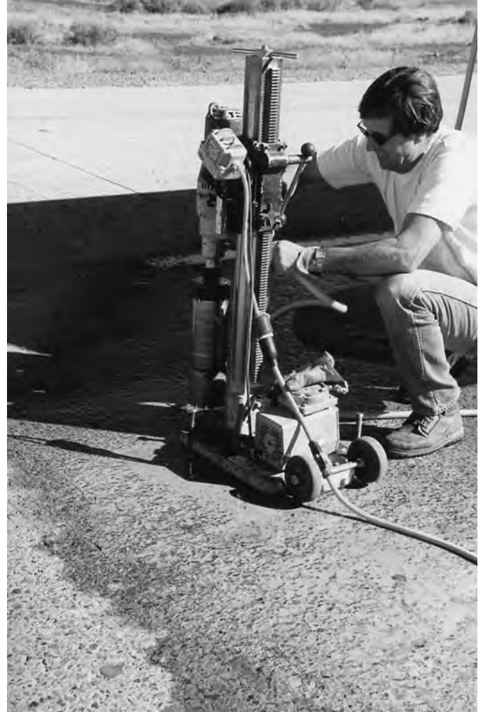
Figure 54. Rented coring rig, Nevada SPS-1.
