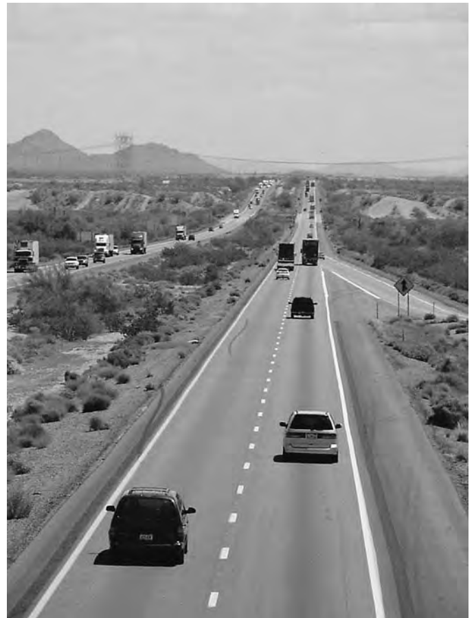
Figure 16. Arizona SPS-2 site.
