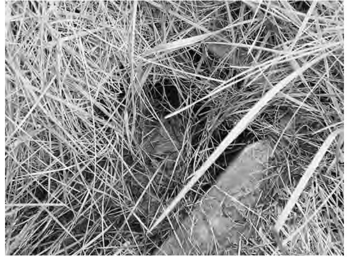
Figure 46. View from above and close-up view of overgrown drainage outlet, Delaware SPS-2.
