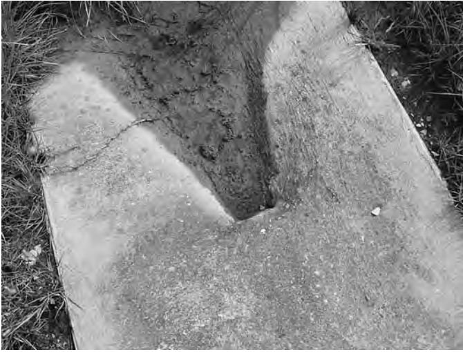
Figure 10. Water and soil at drainage outlet at Alabama SPS-1 site.
