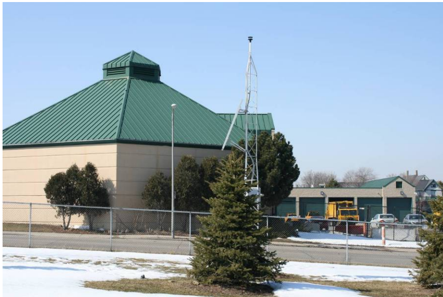
Figure 3.22 Tower Looking West
