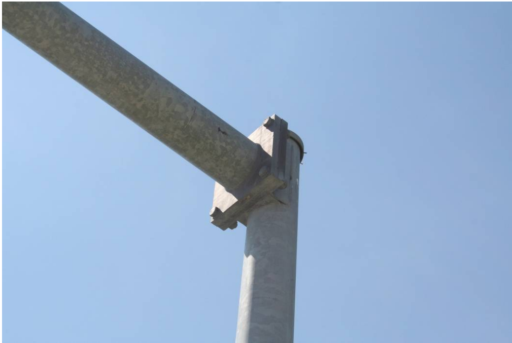
Figure 3.2 Mast-Arm-to-Pole Connection Detail
