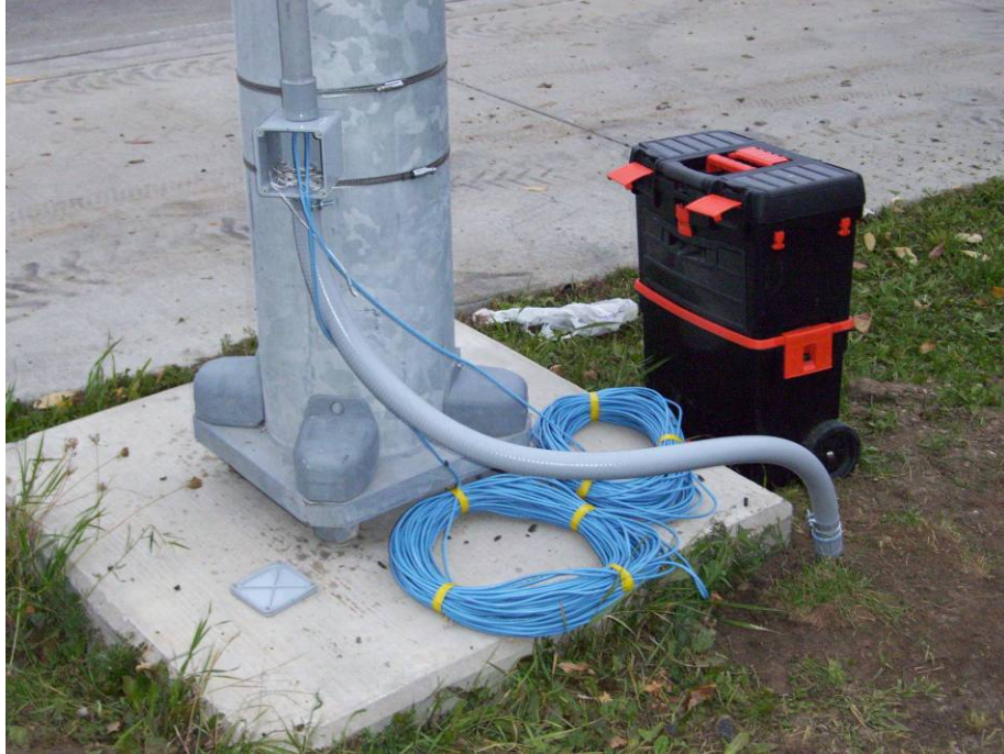
Figure 3.29 Conduit Connection to Sign Support Structure
