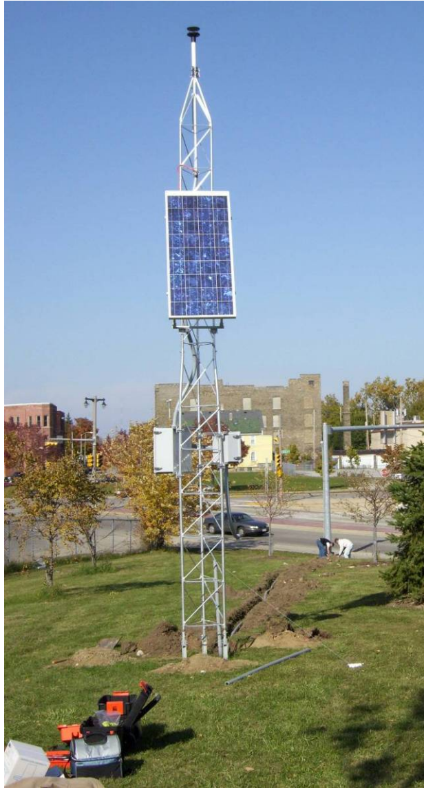
Figure 3.17 Twenty Foot Tall Aluminum Weather Station Tower Installation.
