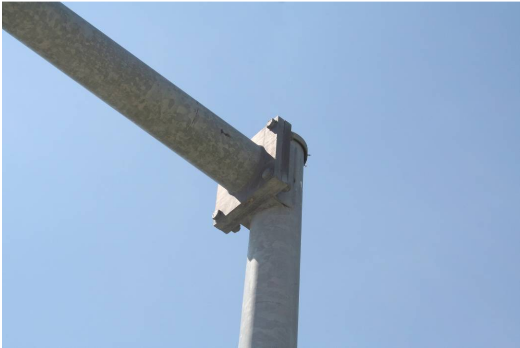
Figure 1.2 Typical Mast-Arm-to-Pole Connection
