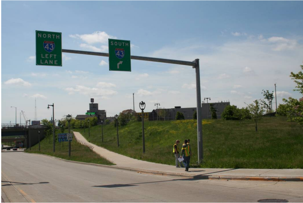
Figure 1.1 Typical Cantilevered Sign Support Structure
