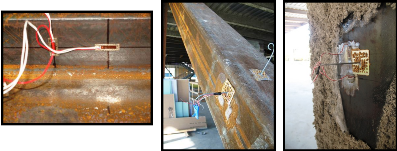
Figures 3.1.10, 3.1.11, 3.1.12: Installed Strain Gauges in the DLC
