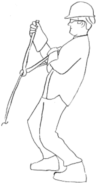
Fig. 4. A line worker cutting a large diameter wire with a manual cutter (EPRI, 2001).
