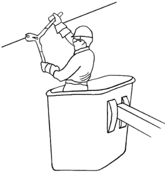
Fig. 3. An overhead line worker crimping a compression connector with a manual compression press from a bucket. Courtesy of EPRI (December 2001).
