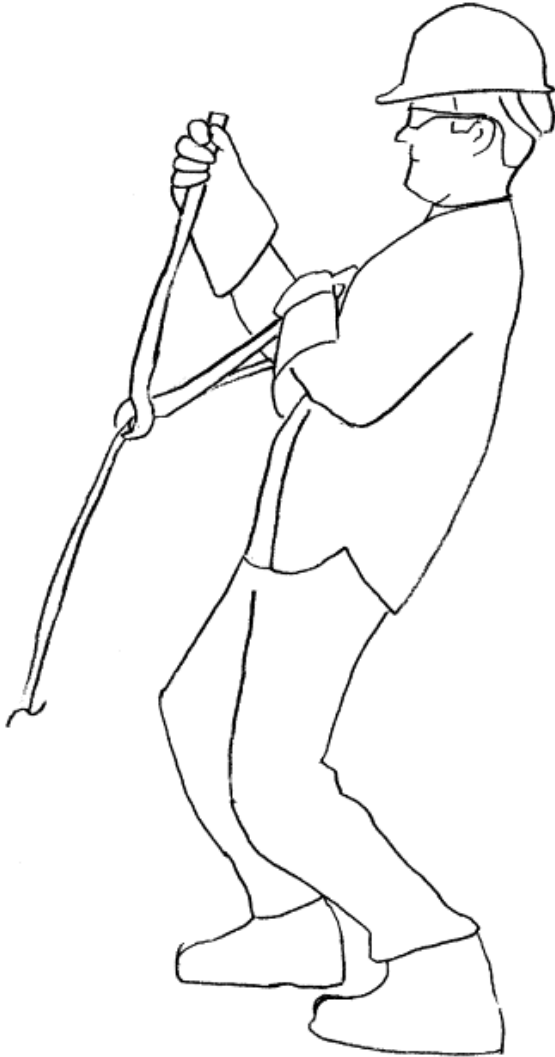
Fig. 5. An underground line worker cutting a wire with a manual cutter. Courtesy of EPRI (December 2001).
