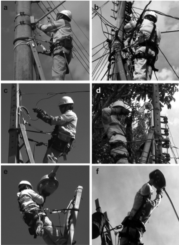
Figure 1. Electrical overhead workers performing three tasks in simulated and field environments. (a) Relay replacement task in simulated environment. (b) Relay replacement task in field environment. (c) Consumer connection/disconnection in simulated environment. (d) Consumer connection/disconnection in field environment. (e) Bulb replacement in simulated environment. (f) Bulb replacement in field environment.
