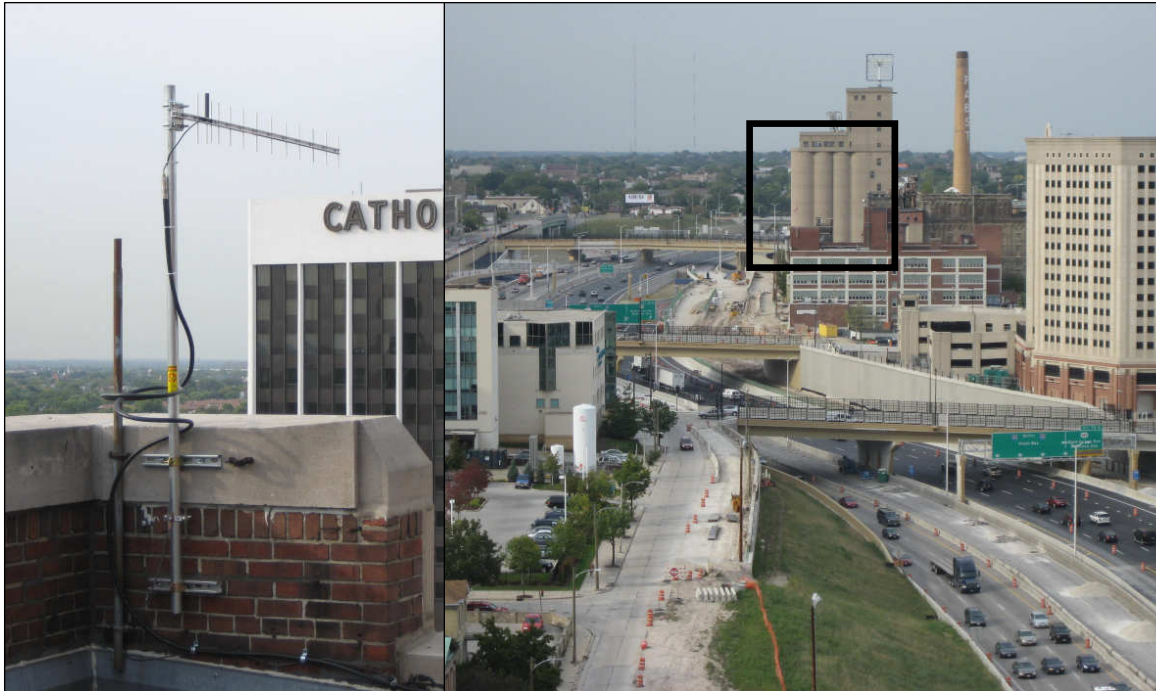
Figure 2-12 - Left: The wireless antenna mounted on the corner of Carpenter Tower Hall at Marquette. Right: View from the antenna location at Carpenter Tower. The test section is located just behind the grain elevators in the highlighted area.
