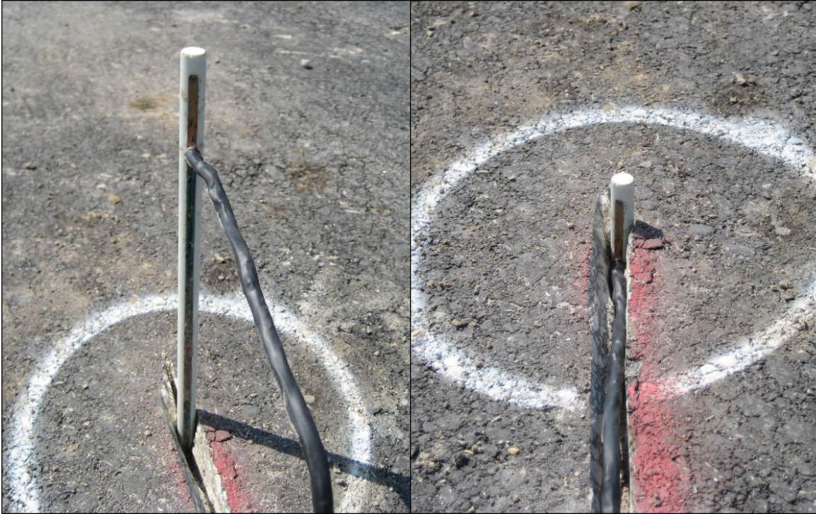
Figure 2-13 - The photograph on the left shows almost the entire length of the temperature probe. The photograph on the right shows the temperature probe fully inserted to its final position. Note that the sensor lead is fitted into its channel, but has not been sealed yet.
