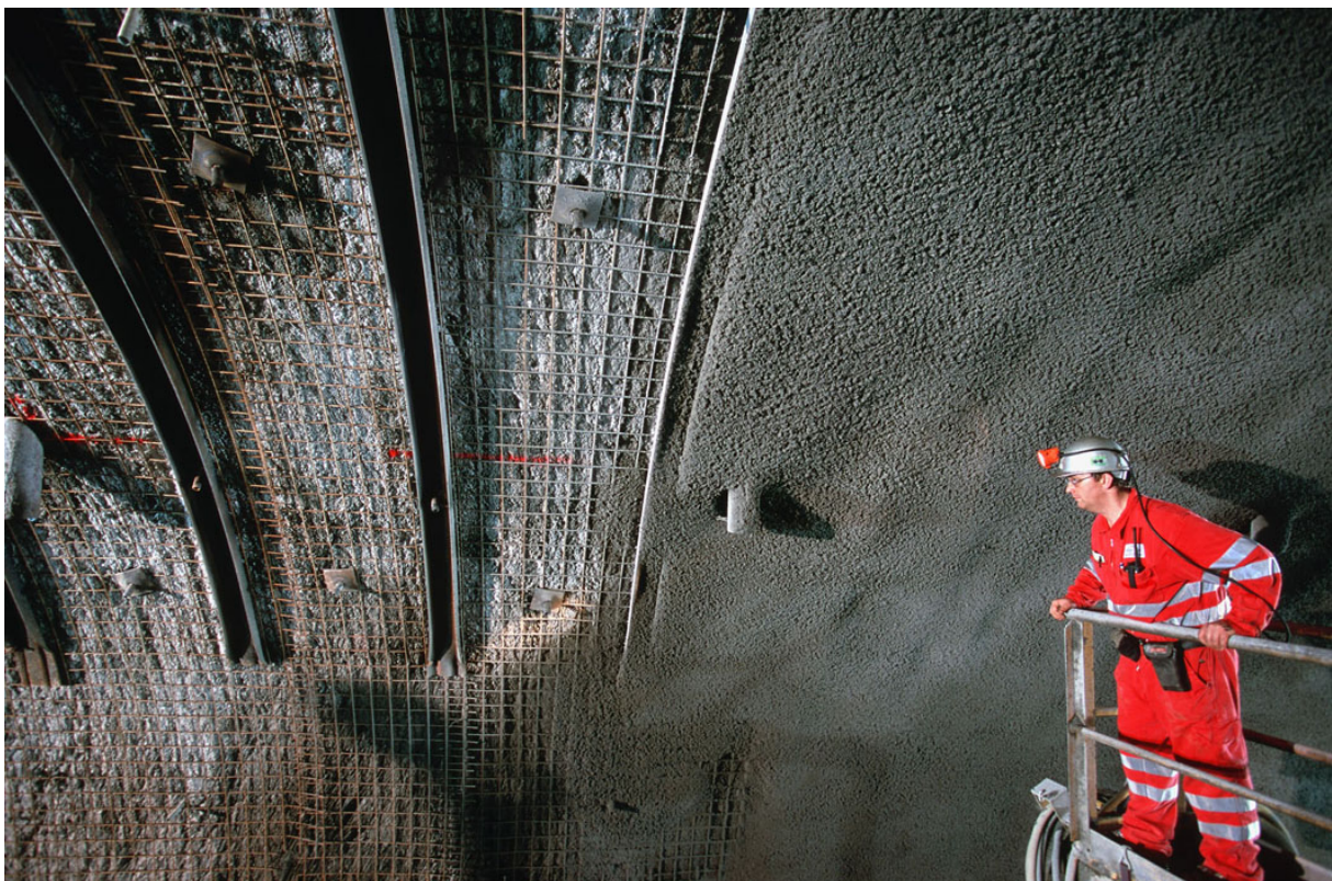
Slika 8: armirana brizgana betonska stena v predoru (vir: http://www.tunneltalk.com )
