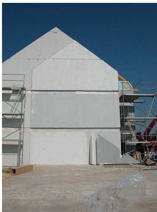
Pic. 4 Gable wall with Multipor
