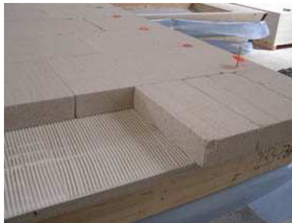
Pic. 3 Glueing of Multipor
