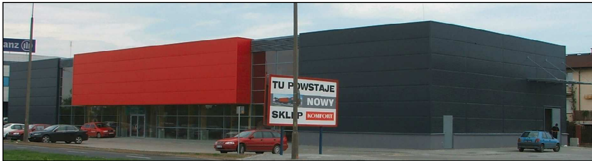
Fig. 5 The building facade
