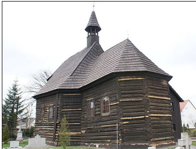
Fig. 3 The walls of the church
