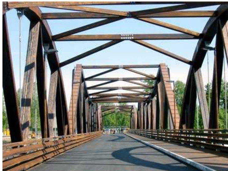
Fig. 7 View of the new Flisa bridge
