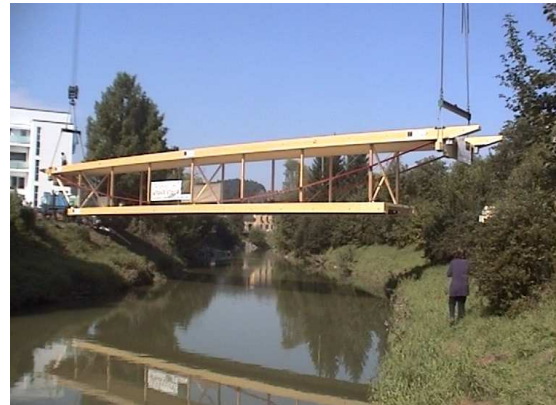
Fig. 6 Assembly of the bridge
