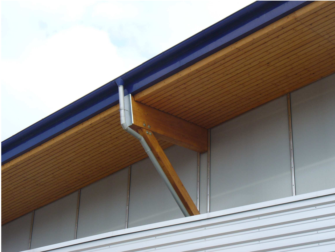
Fig. 11 Detail of protecting timber parts against weathering
