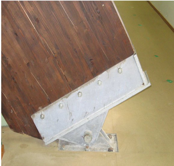
Fig. 10: Connection of the main timber element to the concrete foundation.
