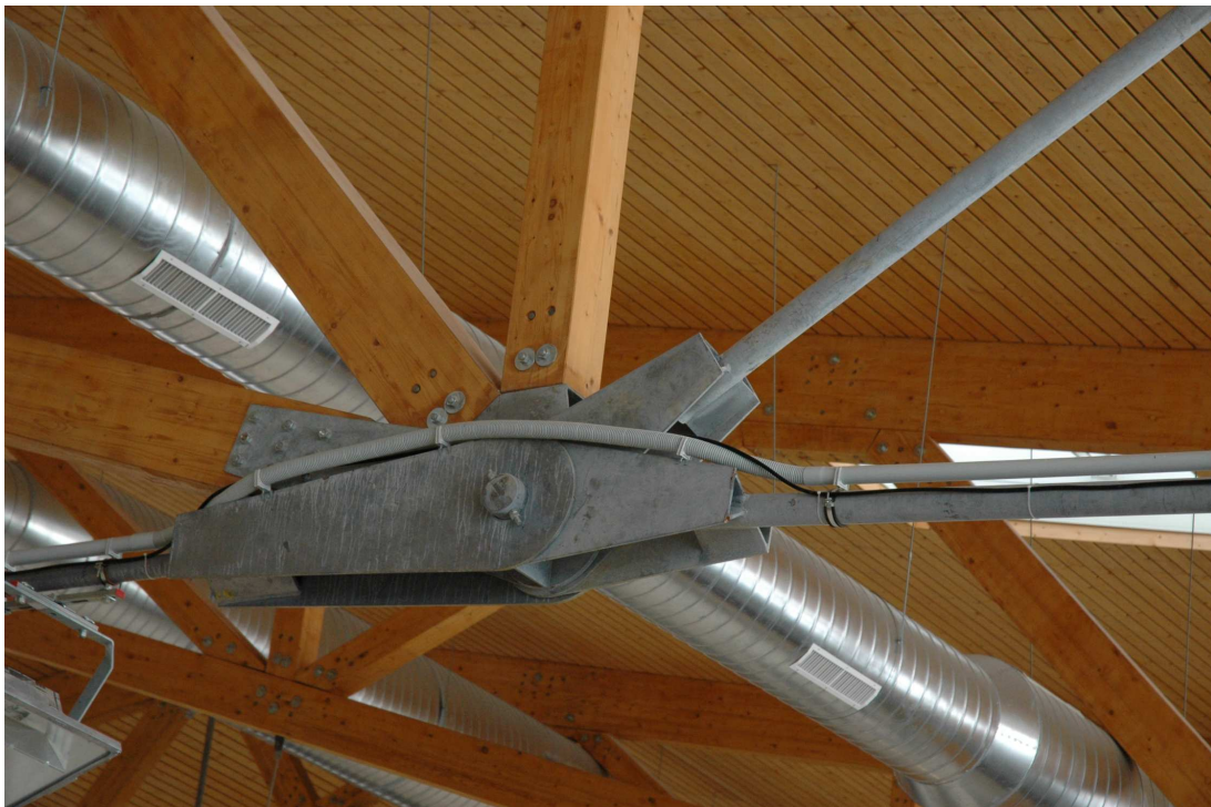
Fig. 10 Detail of timber - steel bars joint
