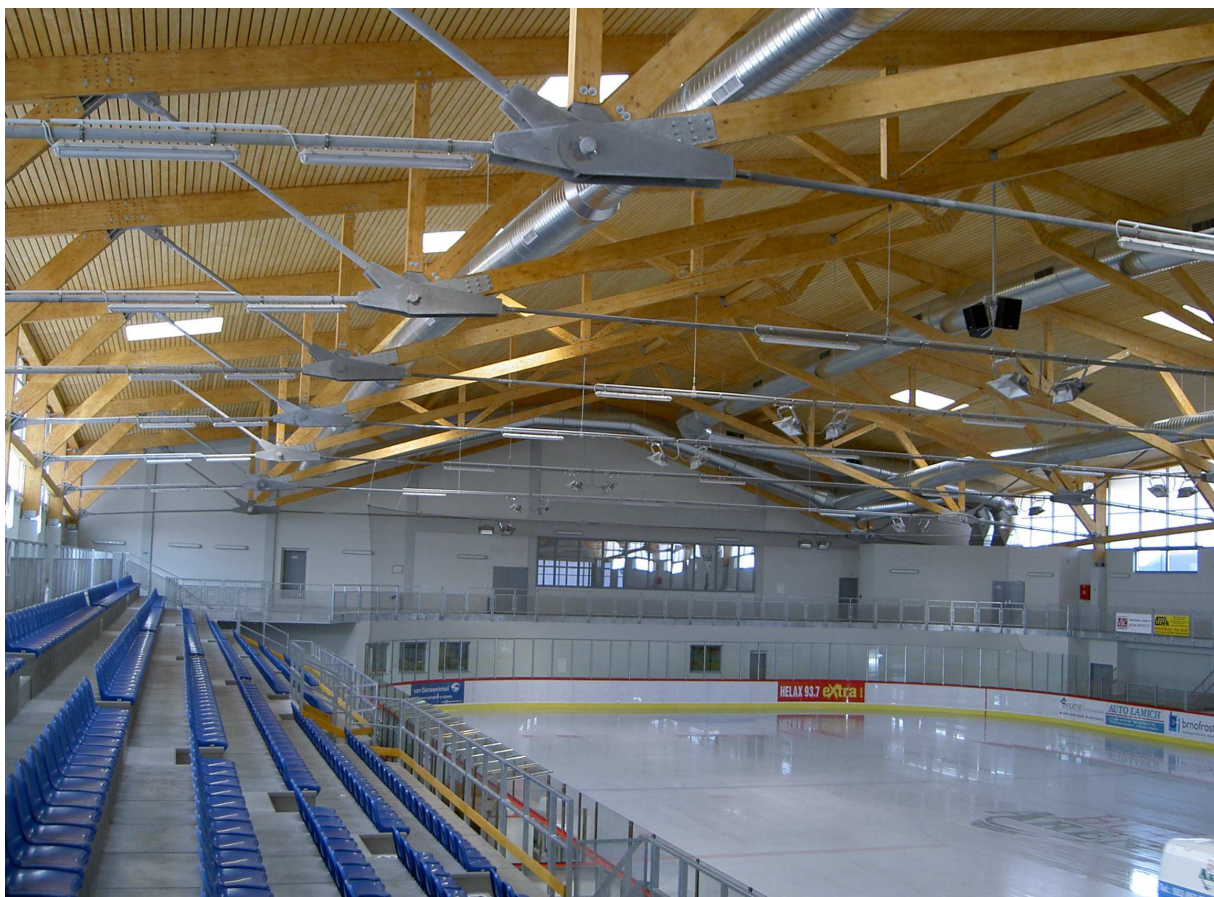
Fig. 2 Bearing system of the roof
