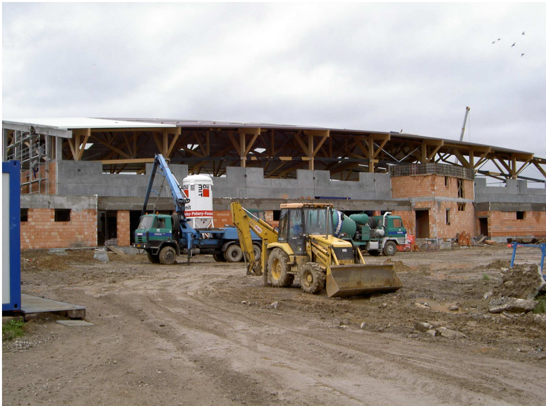
Fig. 9 Erection of the bearing system
