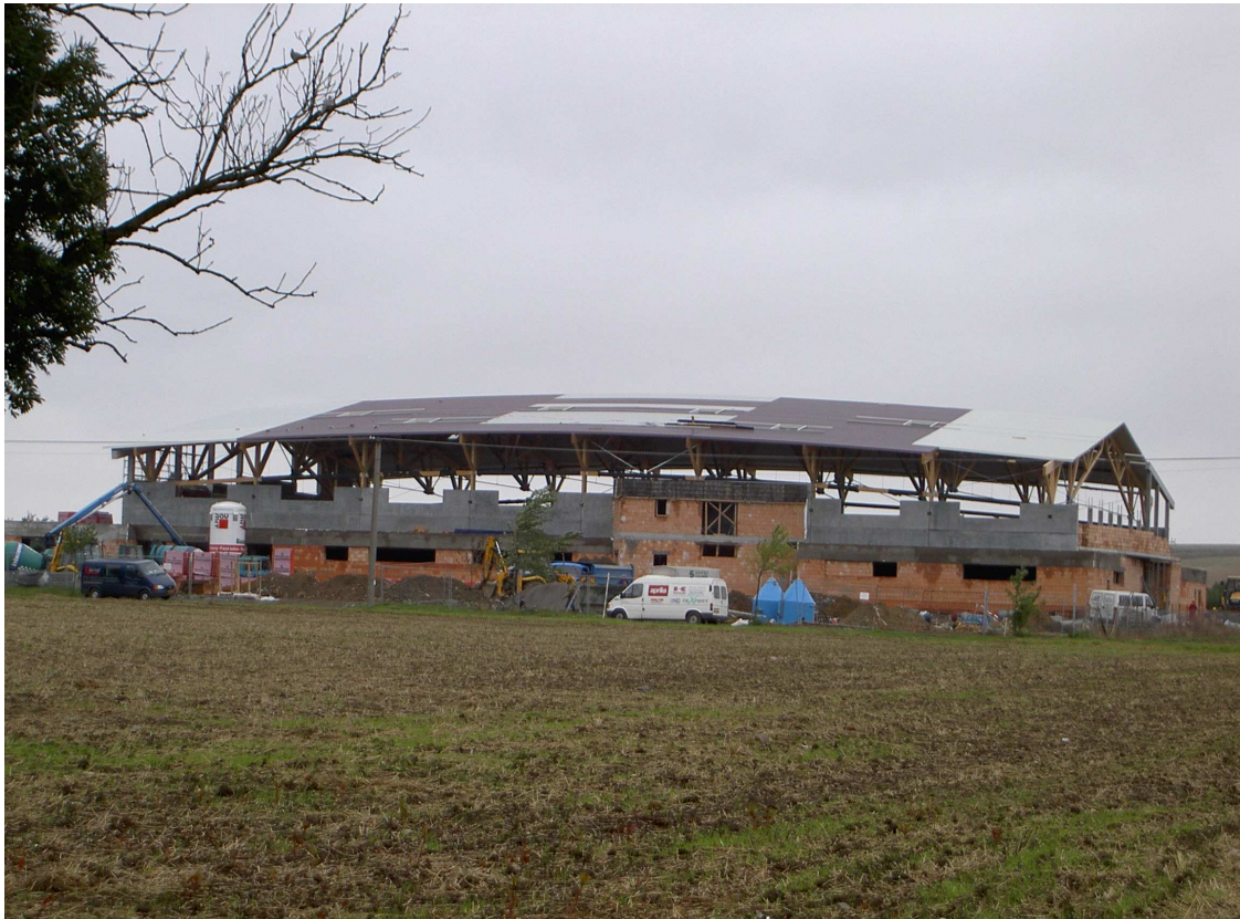
Fig. 8 Erection of the roof
