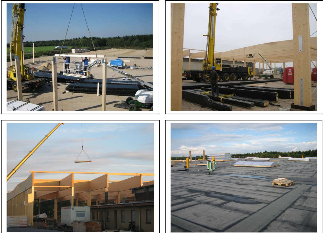
Fig. 4 Erection of the building
