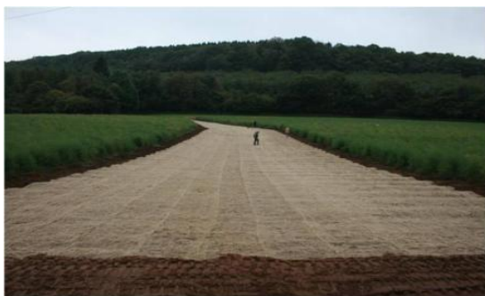
Figure 18: Potential eroded channel ('thalweg') lined with jute geotextile.
