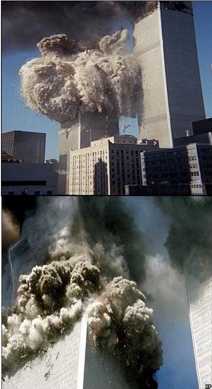
Plate 24: The South Tower (2 WTC) collapsing at 9.59am on September 11, 2001. The North Tower (1 WTC) on the right of the photograph collapses later at 10.28am.
