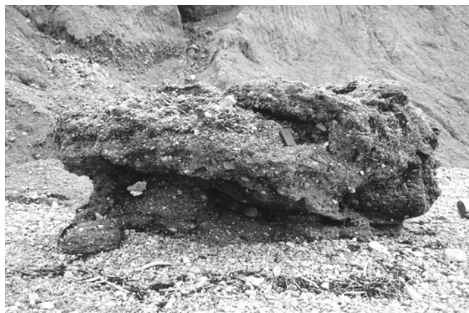
Figure 7. Fallen block of the indurated cobble gravel unit, indicative of a possible rockfall hazard below the cliffs.
