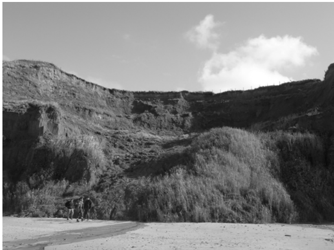
Figure 6. Kettle hole failure in silts at [230650 340955].
