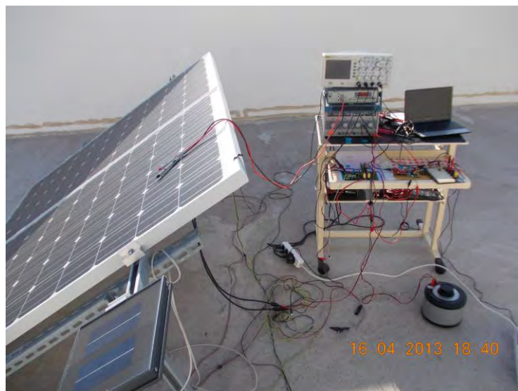
Figure 6.5. EPS PV Lab outdoor measurement bench.
