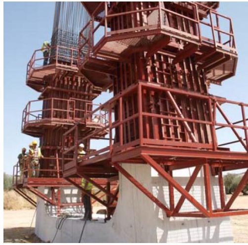
Source: AZVI constructions
