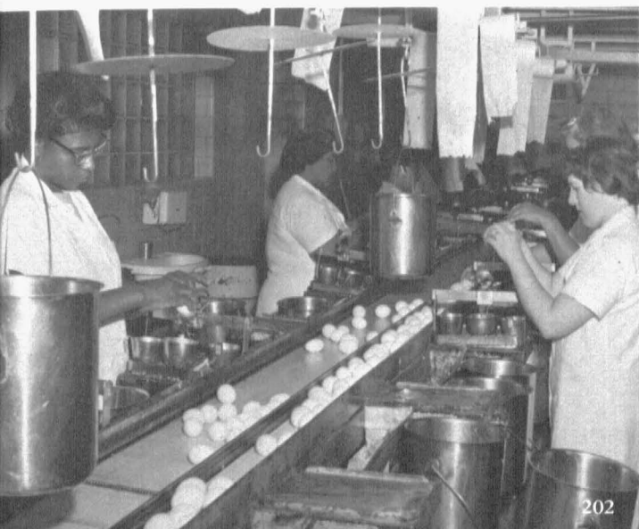
Fig. 203—Egg breaking machine. Note separation of yolks and whites.
