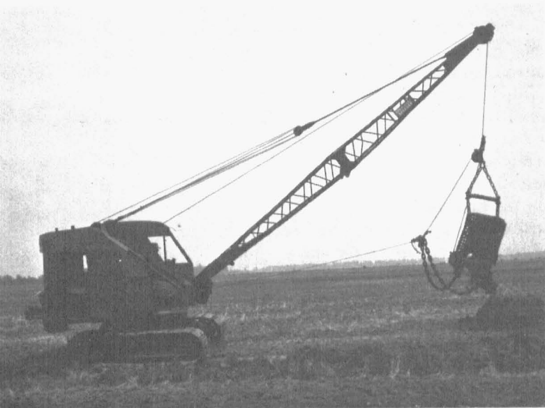
Digging out drainage channel with drag line.
