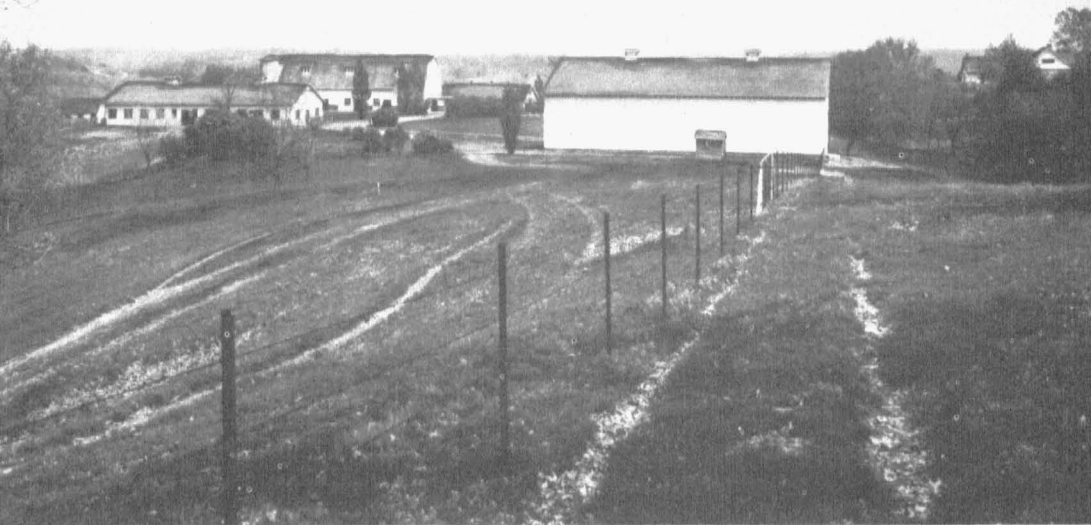
Hatch Farm buildings (left to right): Bull barn, young stock and maternity barn, milking barn and dairy house, hay barn, and residence.
