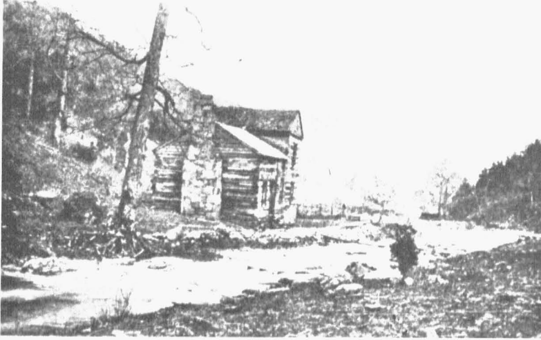
A real pioneer cabin of the eastern mountain region, with its hewn logs, "chinked" with mud or plaster, and its big stone chimney. A stream of water ran nearby. (After Oakley).
