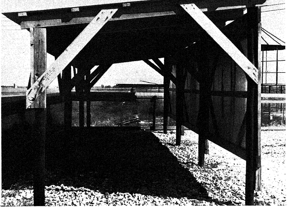
Fig. 13—A structure designed to provide shade for silage in plastic bags. The front panels were on the south side and were removable to permit placing the bags (on pallets) under the structure.
