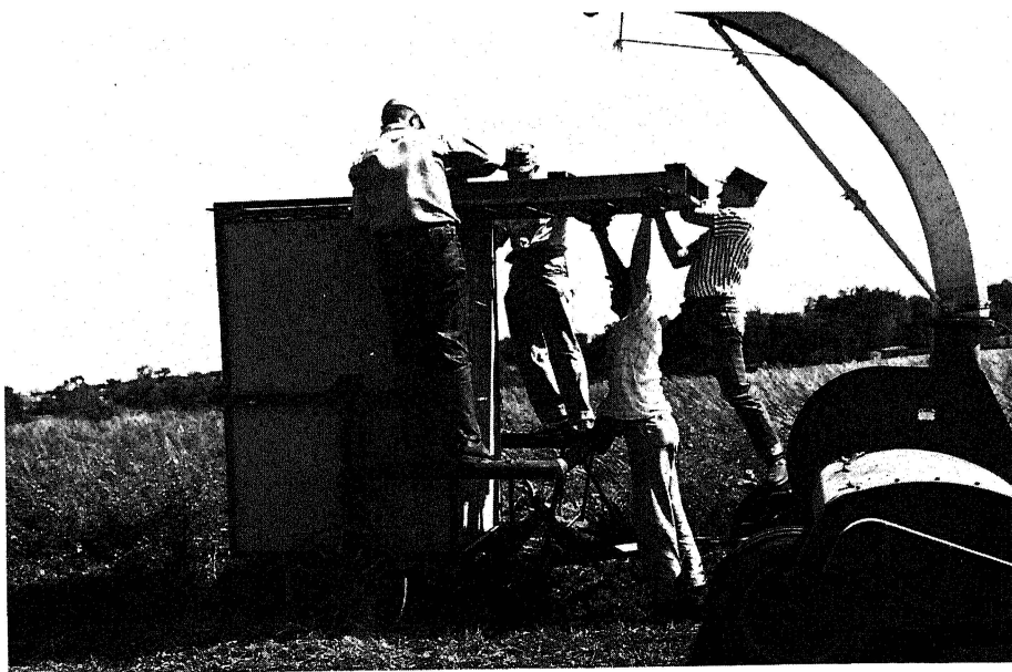
Fig. 2—A 4-ft. x 4-ft. pallet was placed upside down in guide rails above the filled bag.
