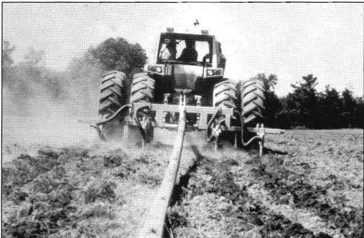
Figure 4. On-site injection units are fed with biosolids pumped continuously from the treatment plant.
