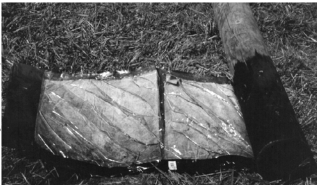
Figure 18. Example of an external supplemental preservative system used to arrest external decay at ground line.
