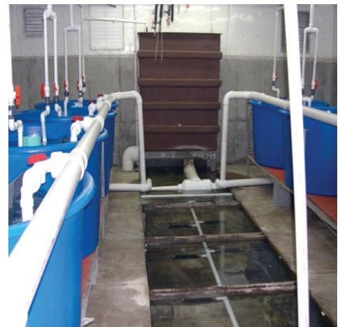
Figure 10. The waste pit allows solids to settle and be removed to the lagoon through a drain at the end of the pit.
