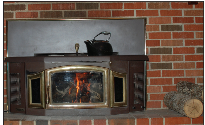
Figure 1. A fireplace insert can greatly improve the efficiency of a conventional fireplace.
