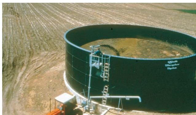
Figure 3. Circulation with a high-volume pump agitates the contents of this glass-lined steel tank.
