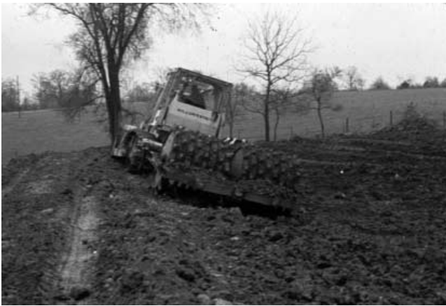
Figure 2. A sheep's foot roller is commonly used to compact the clay seal during construction of a lagoon.
