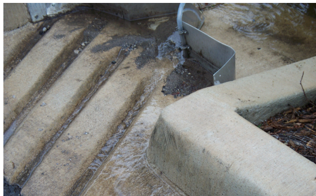
Figure 25 Grooves at Inlet
