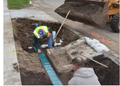
Figure 64 Photo of Bioretention Cell
