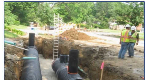
Figure 63 Photo of Bioretention Cell with Smart Drain® (Source: Dods, 2012)
