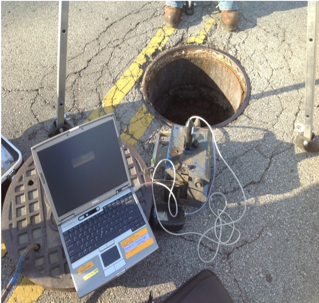
Figure 2-1 Air monitor and computer connection for flow meter data collection
