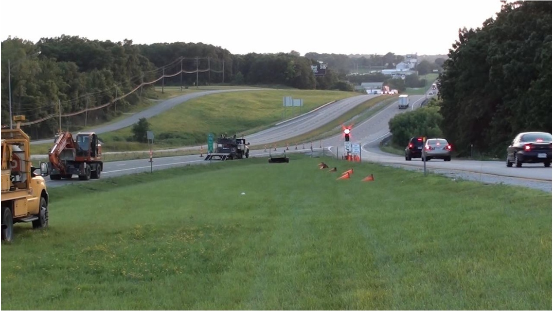
FIGURE 3.6 I-70WB @ mile marker 131, three-head signal.
