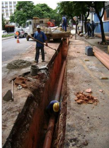
Figure 2- 1: Steel Pipe Installation (Wikipedia, 2009)
