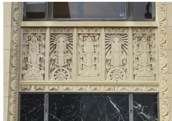
Figure 3.5. Exterior of the Kansas City Power and Light Building featuring Art Deco elements like curlicue stylized fountains and radiating sunbursts.
