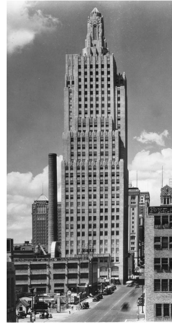
Figure 3.3. The Kansas City Power and Light Building, ca. 1935, Robert Askren Photograph Collection (P35), box 2, folder 10, no. 4, Missouri Valley Special Collection.
