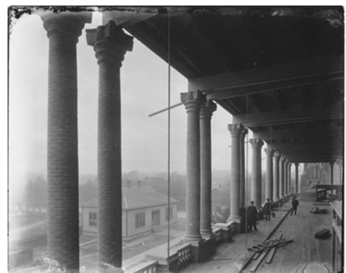
Figure 2.3. View showing the scale of the upper loggia of the first Convention Hall. General Collection (P1), Convention Hall, Number 4, Missouri Valley Special Collections, Kansas City Public Library, Kansas City, MO.
