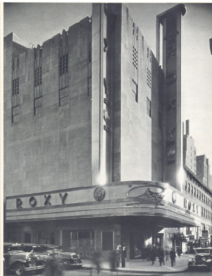
Figure 4.9. The RKO-Roxy Theater, New York City. Photo taken by Browning Studios, from American Architect , no. 2614 (December 1932): 41.
