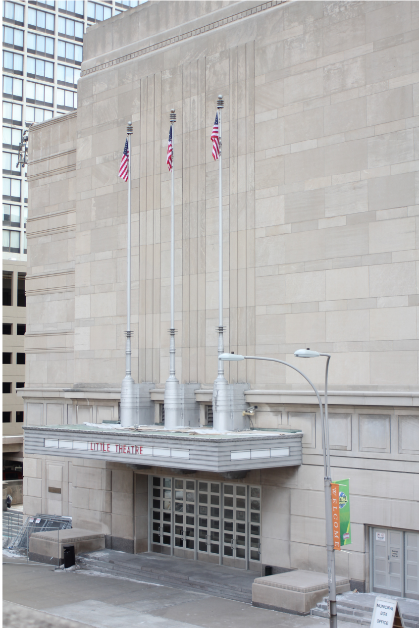
Figure 4.11. Marquis and flag poles along 13th Street above the entrance to the Little Theater in the Municipal Auditorium, Kansas City, MO. Photo by Jayson Gray.
