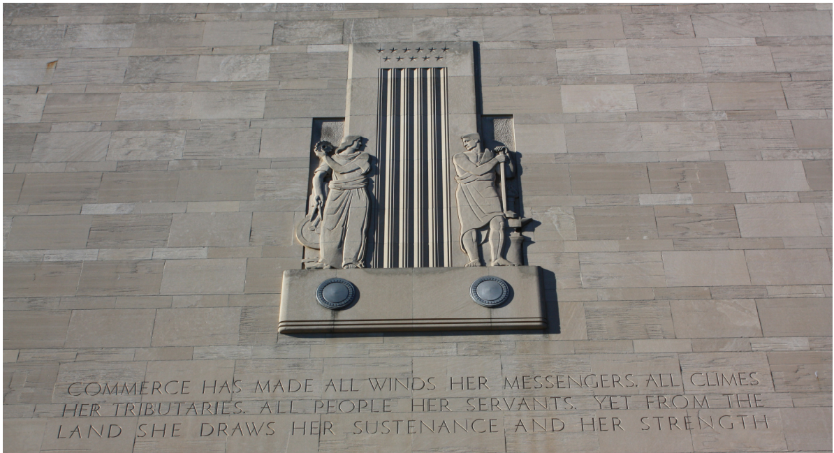
Figure 4.23. Albert Stewart, designer, and H. F. Simons, carver, Industry and Commerce , plaque on the south façade of the Municipal Auditorium, Kansas City, MO.
