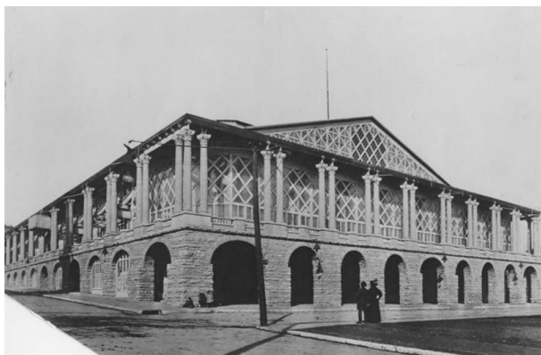
Figure 2.2. The first Convention Hall. General Collection (P1), Convention Hall, Number 5, MO Valley Special Collections, Kansas City Public Library, Kansas City, MO.
