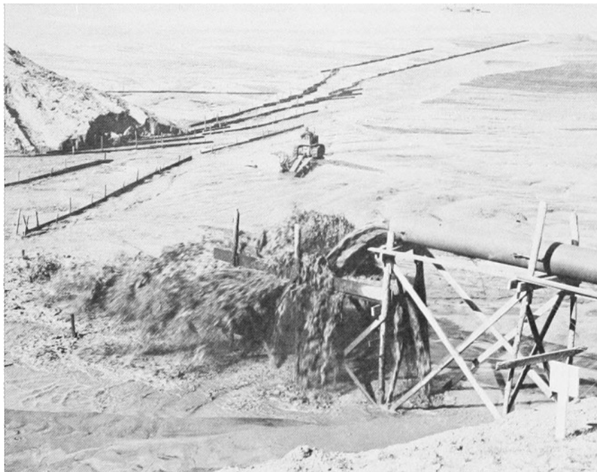
Figure 12 - Hydraulic Fill Being Discharged (Corps of Engineers 1985)
