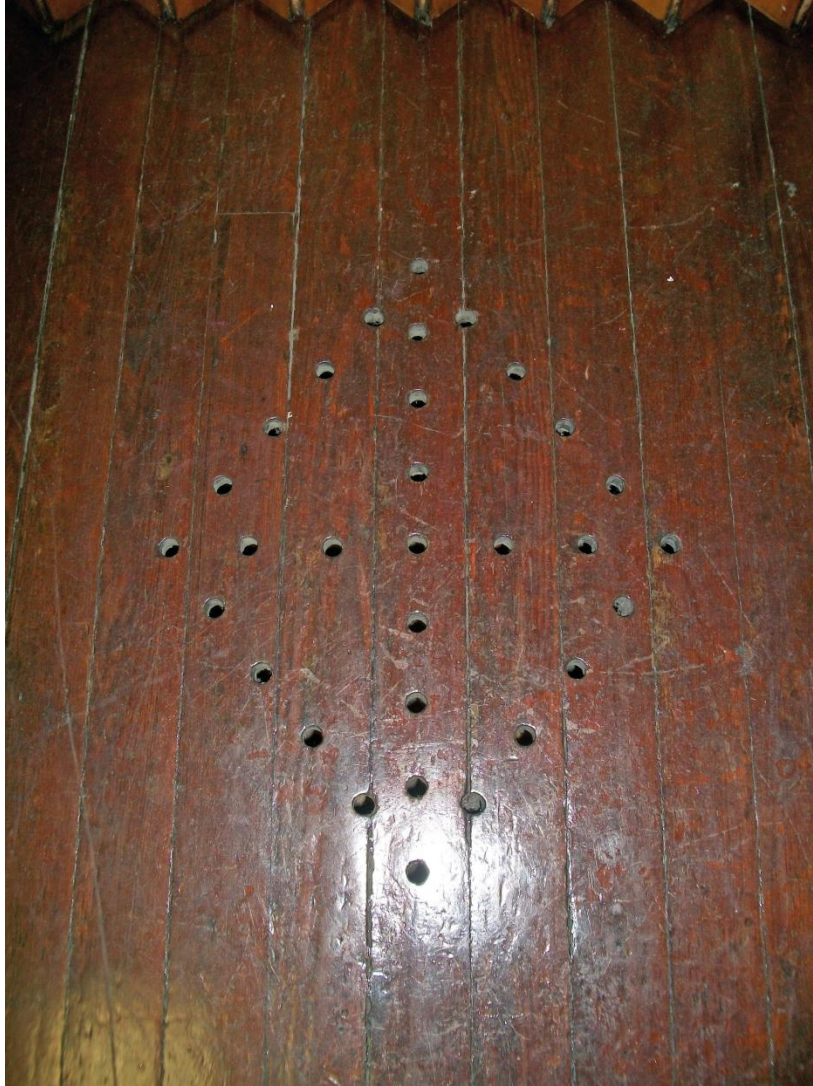
Figure 2-20. Basement floor of First African Baptist Church with diamond shaped Congo Cosmogram for ventilation of the space beneath. Photo by L. Clifton-James 04/01/10.
