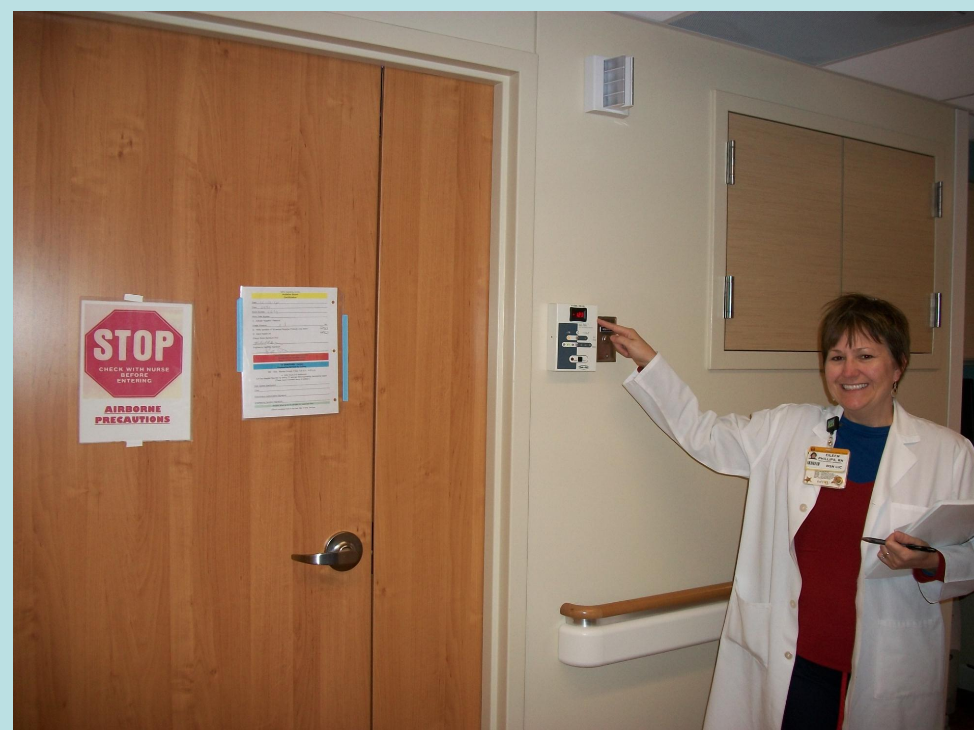
Figure 1: Private room with negative air pressure at the University of Missouri Hospital
