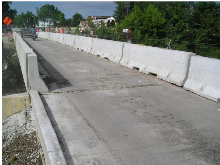
Figure 1-1 Bridge and bridge approach slab
