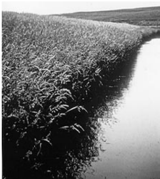
Figure 2. Fescue, reed canary or other heavy grass may be sufficient to protect the dam from wave action.
