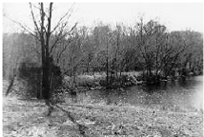
Figure 5. Don't allow trees and brush to grow on the dam or in the emergency spillway.
