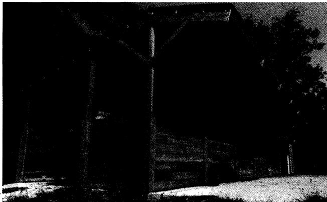
The Swaffer composter is a pole-type structure with monsope, rafter-type roof and a short overhang.
