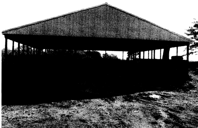
The Ball composter is a pole-type structure with open sides and a wood-truss roof.
