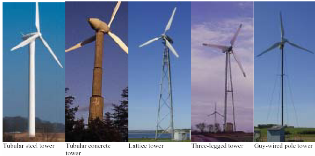
Figure 2.23 : Various tower structures
