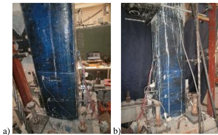
Figure B.45 : a) North, and b) South view of X26-M-CFRP1 after -3.00% mm drift ratio.
