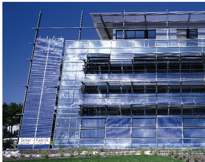
Figure 4.8 : PV-shading device application [47]
