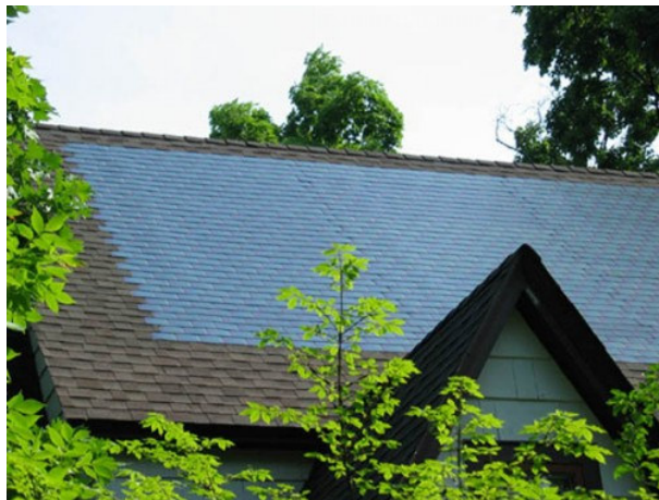
Figure 4.5 : PV roof shingles application [44]
