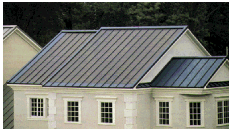
Figure 4.6 : PV metal roof application [45]
