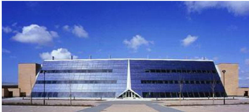
Figure 4.15 : Solar Office Doxford International [52]
