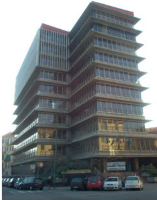
Figure 5.2: ATC Office Building, Turin [28]
