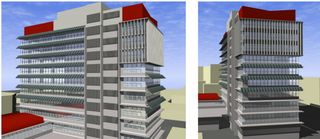
Figure 5.4: Rendering of ATC Building with Photovoltaic Panels - South west and South east Façade [25]
