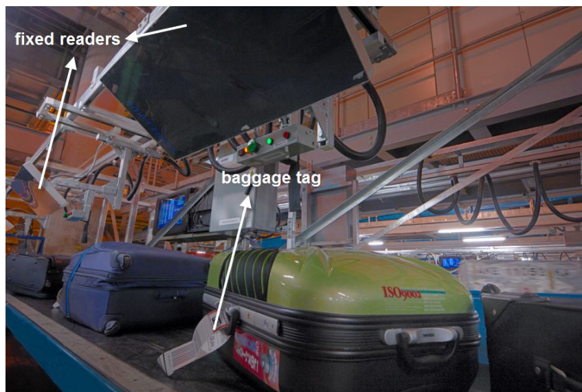
Figure 3.7 : RFID-enabled baggage handling system at the HKIA (Url-9).
