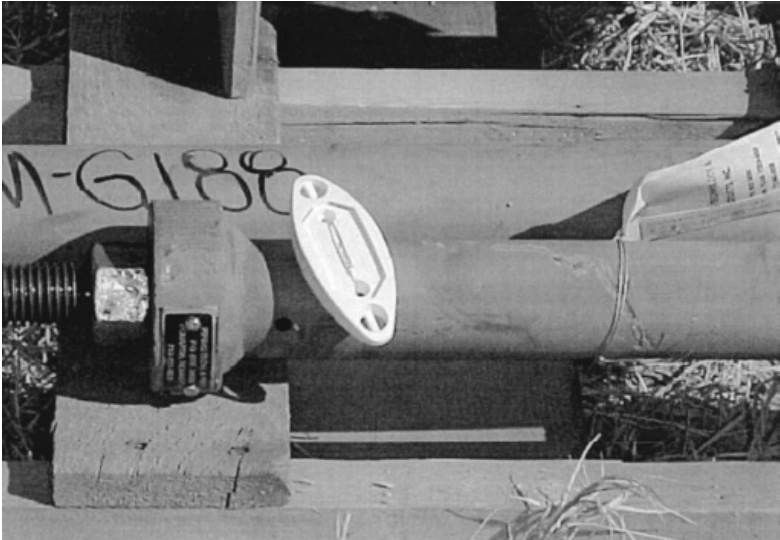
Figure 3.3 : Passive RFID tag attached to pipe support (Jaselskis and Misalami, 2003).
