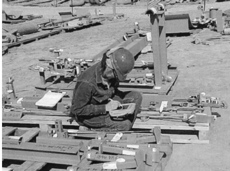
Figure 3.4 : Worker receiving pipe support using RFID approach (Jaselskis and Misalami, 2003).
