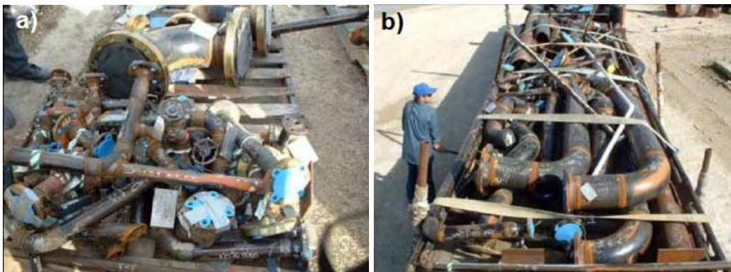
Figure 3.1 : (a) Pipe spools attached with RFID tags and (b) loaded on truck for shipment to job site (Song et al. 2006a).
