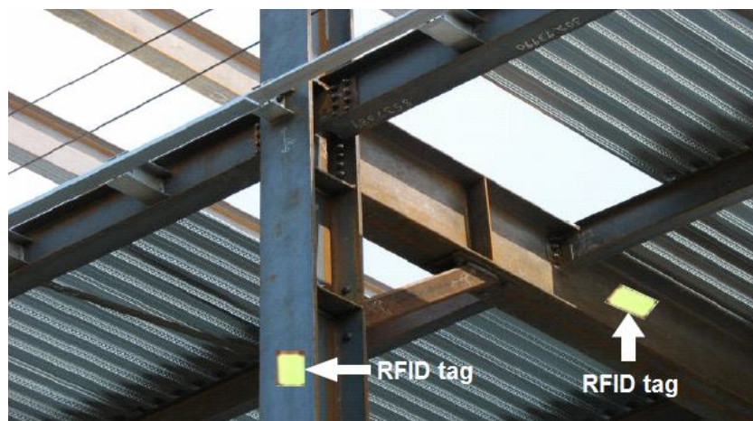
Figure 3.6 : RFID tags attached to structural steel beams and columns (Wenfa, 2008).
