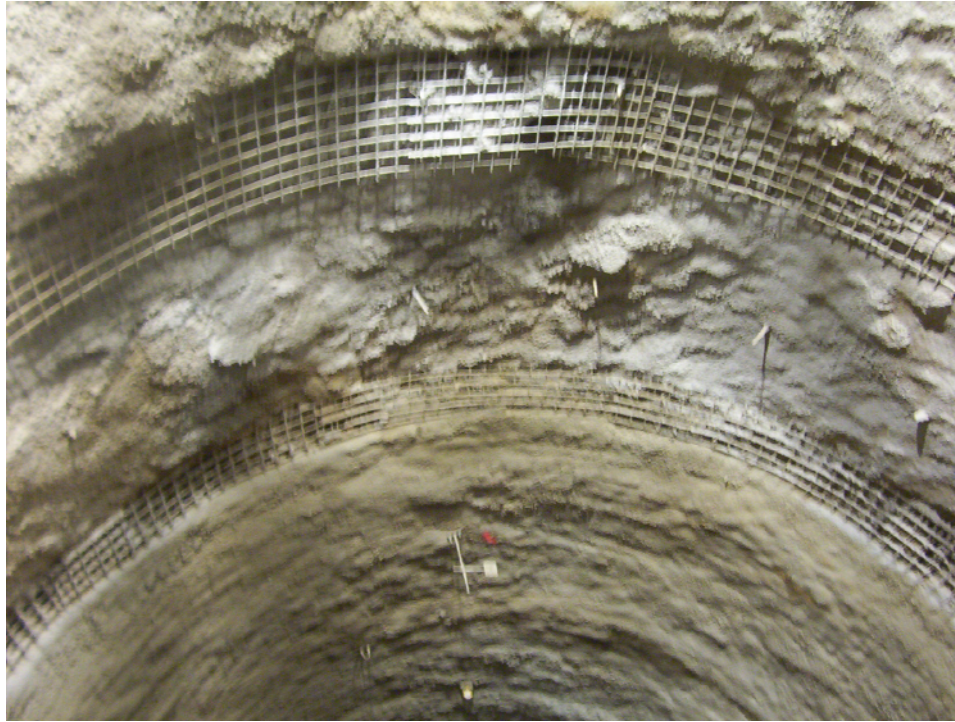
Figure 2.5: Elements in NATM (Wire mesh, Shotcrete, bolts)
