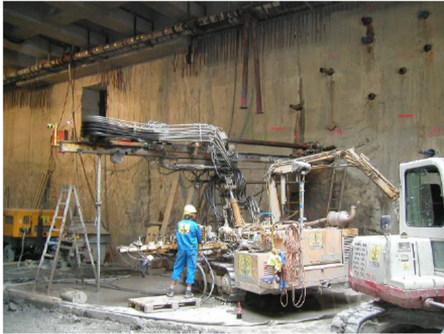
Figure 5.9: Drilling of boreholes of freezing pipes
