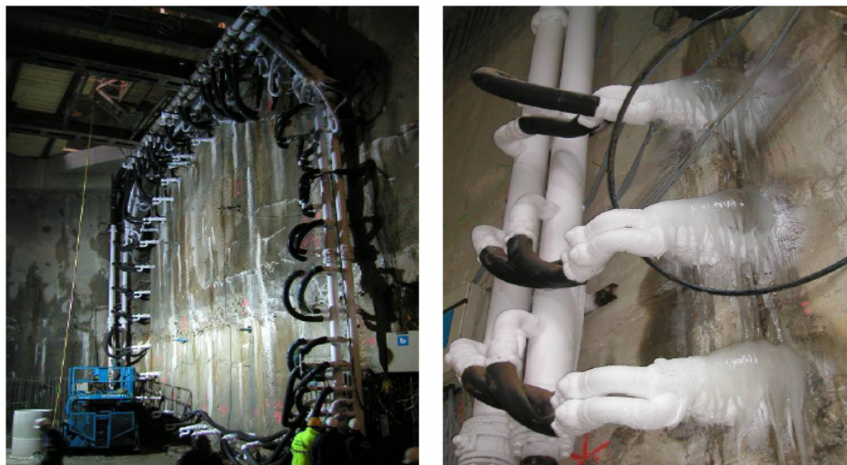
Figure 5.11: Freezing process has begun
