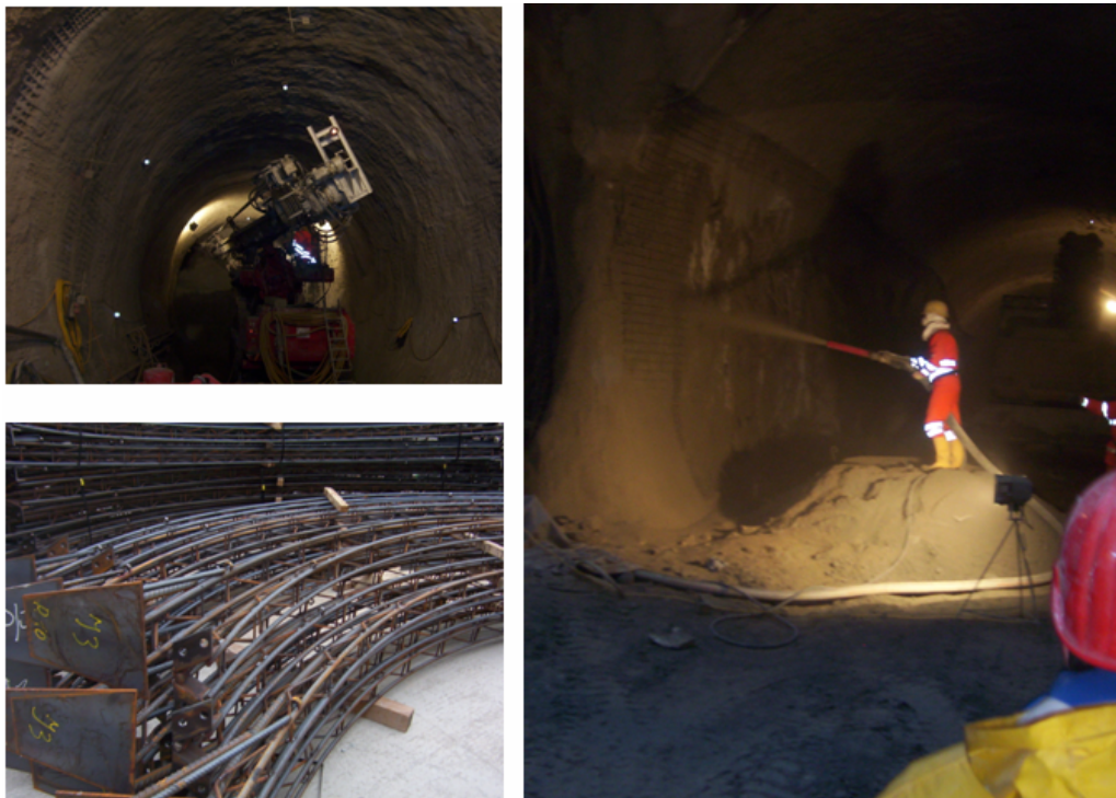
Figure 2.6: NATM tunnelling in U2, Vienna
