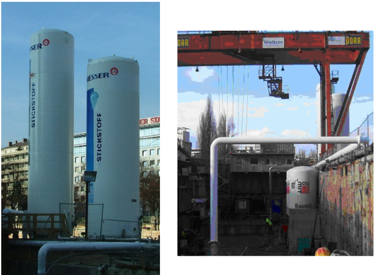
Figure 2.4: Cooler Supplier (left) and connections to the site (right)
