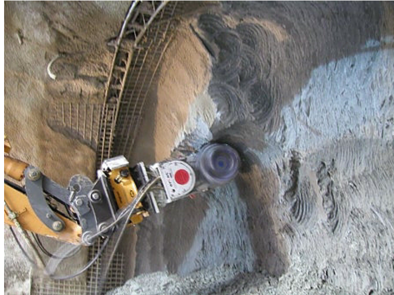
Figure 5.12: Excavation in the Tunnel
