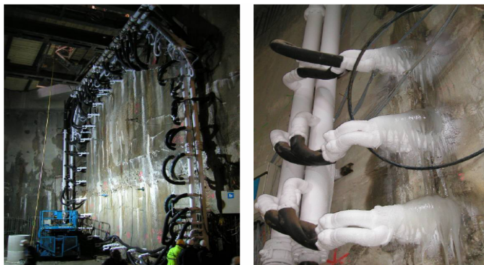
Figure 5.11: Freezing process has begun
