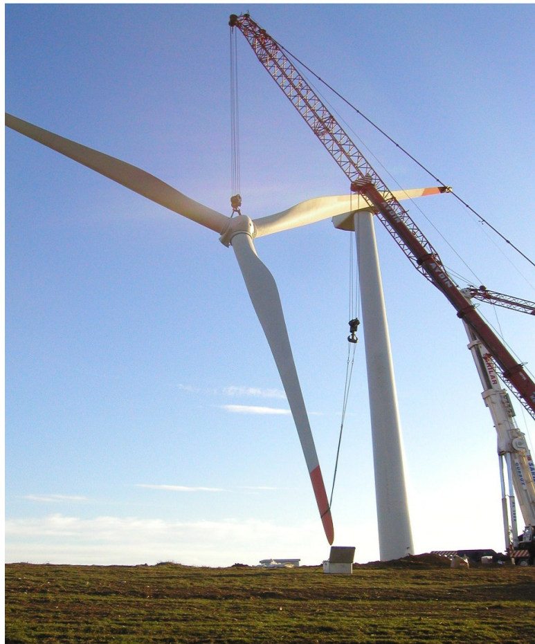
Figure 2.2 Wind Turbine Installation Work
