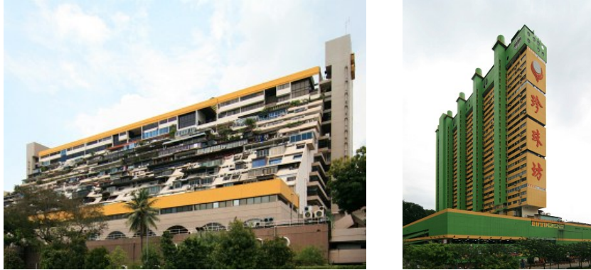
Figure 3.20 : Gold Mile Singapore a.k.a. Woh Hup Complex by William Lim, Gan Eng Oon and Tay Kheng Soon and The People's Park Complex in Singapore by William Lim, Tay Kheng Soon (Url-041).
