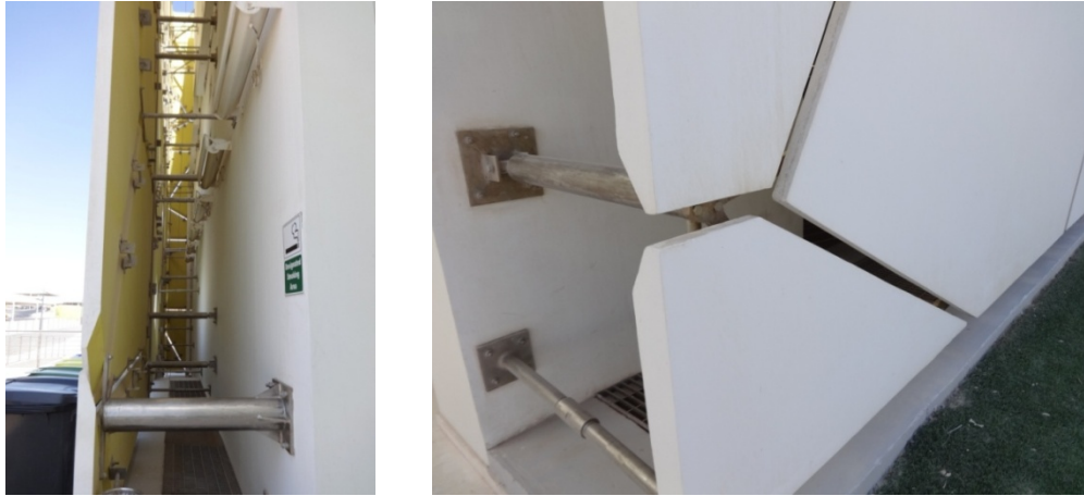
Figure 4.70 : Facade structure (Author).
