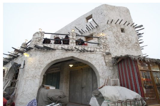
Figure 4.30 : Traditionally built roofs of dangeel wood (Url-093) (Url-094) (Url-095).
