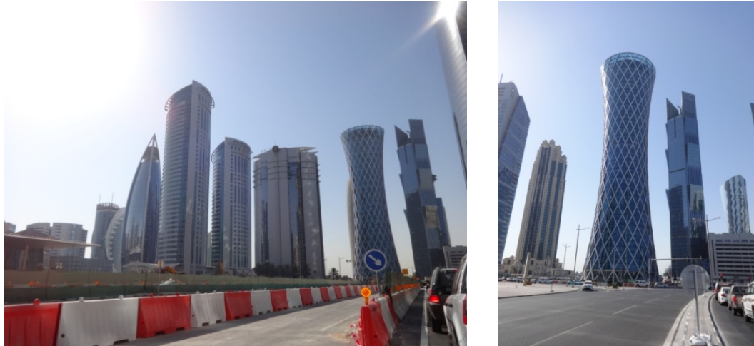
Figure 4.11 : External view in relation to other buildings around (Author).
