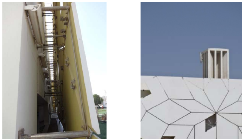
Figure 4.72 : Double wall facade and the wind towers (Author).
