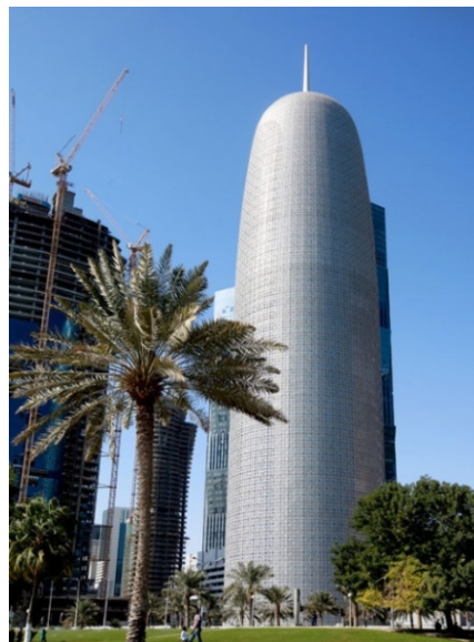
Figure 4.34 : Doha Tower in Qatar (Url-098).
