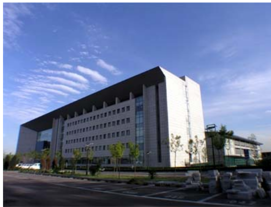
Figure 3.24 : Industrial and Commercial Bank of China Data Centre in Beijing by Tao Ho (Url-046).
