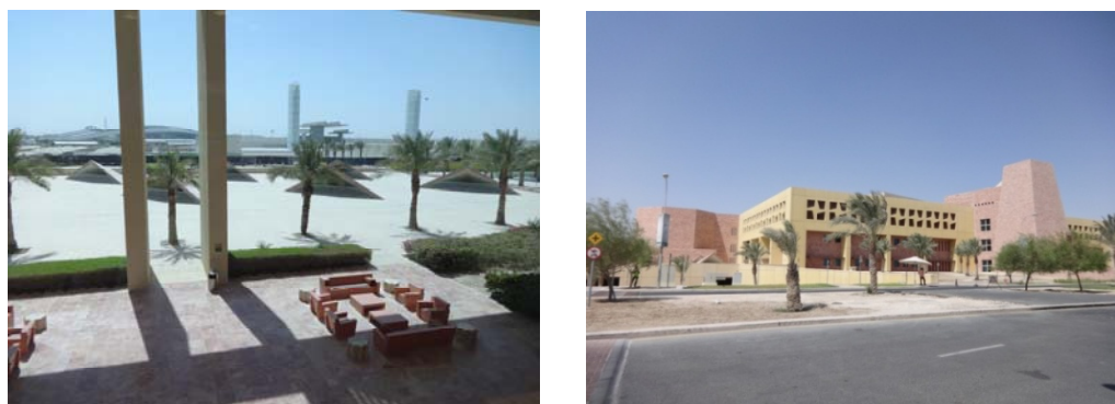
Figure 4.57 : Exterior views of the building (Author).
