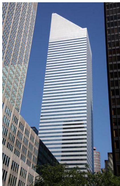
Figure 2.14 : Citicorp Center, Hugh Stubbins and Associates, 1977
