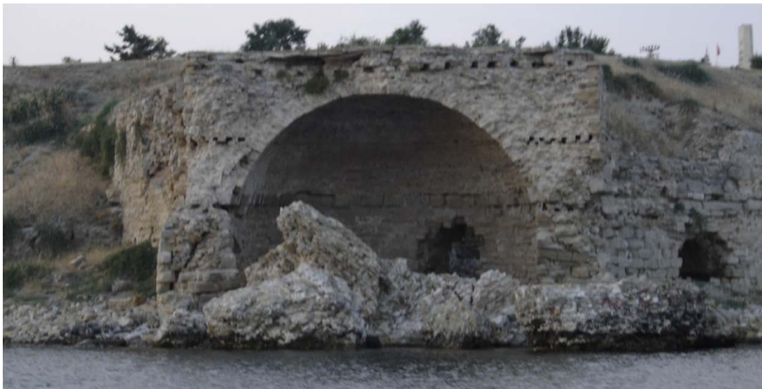
Figure 2.8 : General view of South Tower[10].
