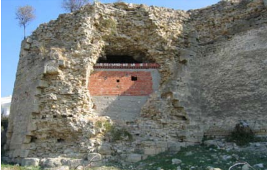
Figure 7.11 : Brick wall built to the window cavity of North Tower [10].
