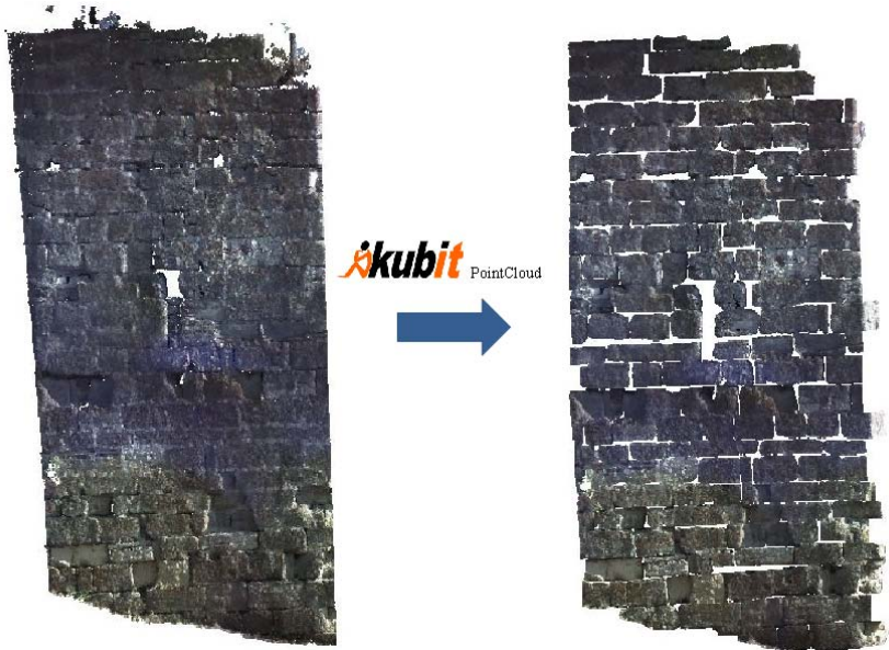
Figure 4.4 : Segmented stones on façade 4 of the North Tower.
