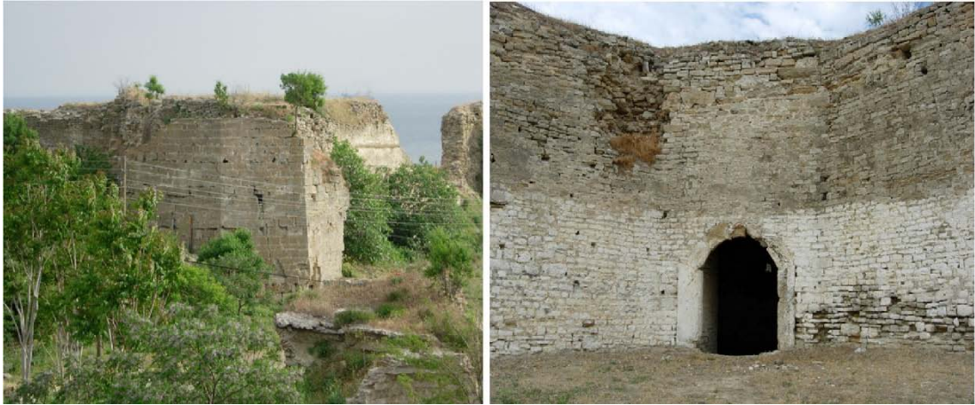
Figure 7.10 : View from the North Tower [10].
