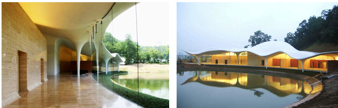
Figure 6.24 : View of concrete roof from inside and outside (Url-171, Url-172).
