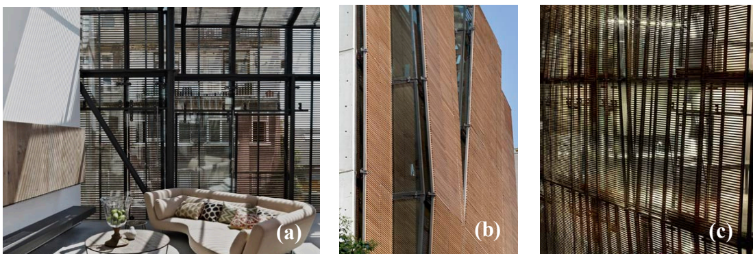
Figure 6.9 : (a)Wooden tulle as sunscreen (Url-147). (b)Glass facets enhancing visual contact (Url-147). (c)Wooden tulle as privacy screen (Url-147).
