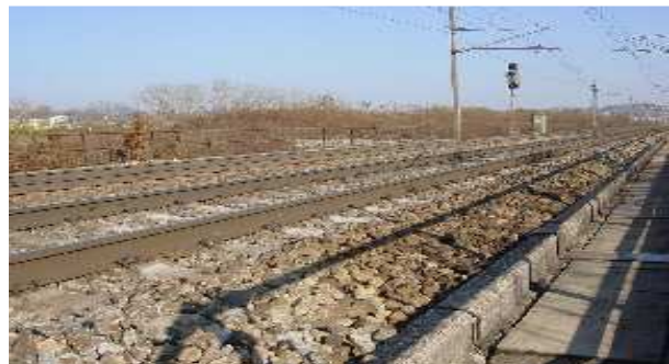
Figure 6: View of the railway track over the bridge.
