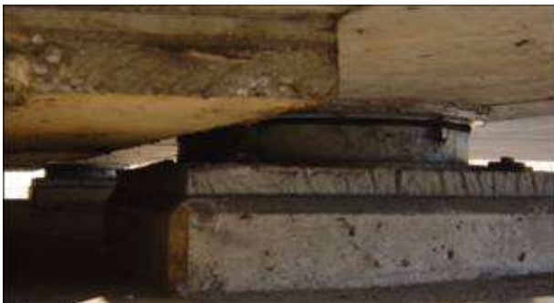
Figure 5: Bearings supports.
