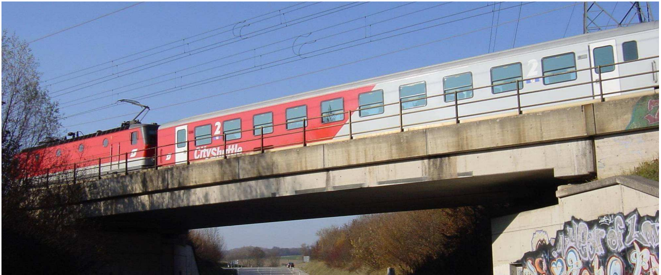
Figure 4a: General view of the bridge.
