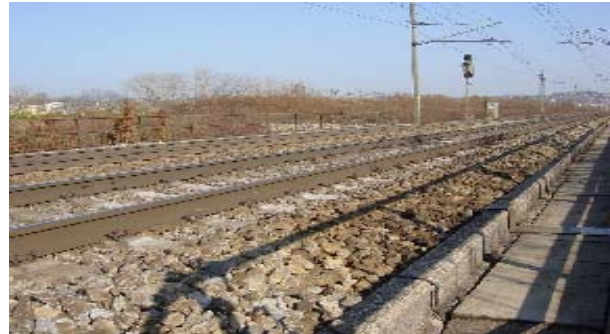
Figure 7: View of the railway track over the bridge.
