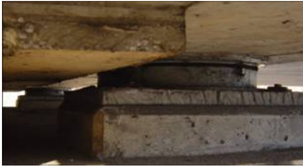
Figure 6: Bearings supports.
