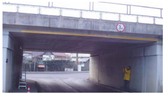
Figure 2–Bridge7 (filled beam): general view
